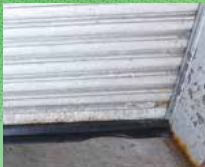
Up-and-over garage doors, and roller shutters can be proofed along the ground with a flexible ‘rubber’ seal.
