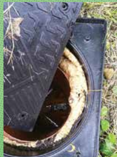
Expanding foam should be rarely employed, as it’s easily nibbled away and can degrade over time. It can be used to provide a first-aid measure, where more permanent works are scheduled at a later date. It is useful as a void filler to allow an outer plug of thick mortar.
